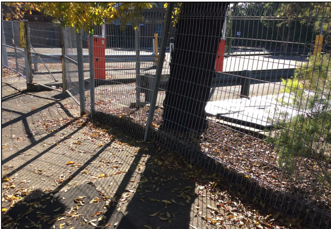
Image 17: Damaged footpath from trees within the site
