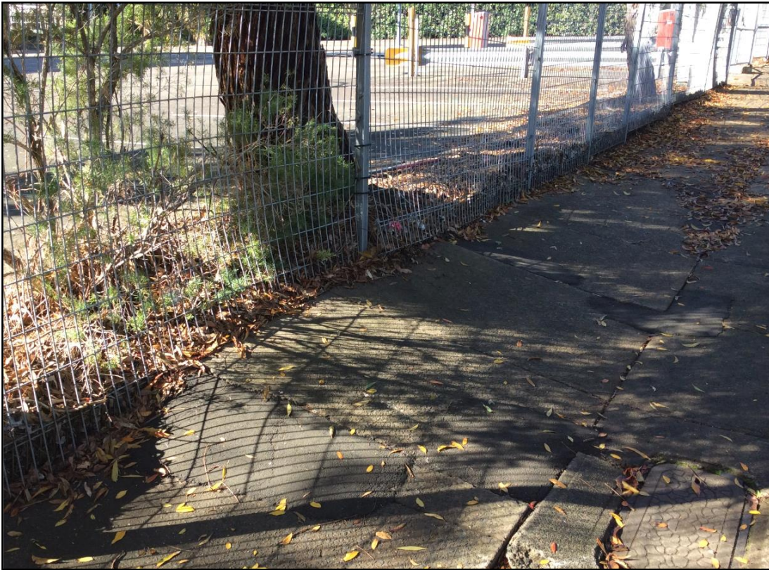
Image 16: Damaged footpath from trees within the site
